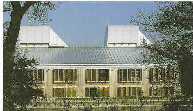
Fig 2.02 Elevational detail showing external timber shutters
