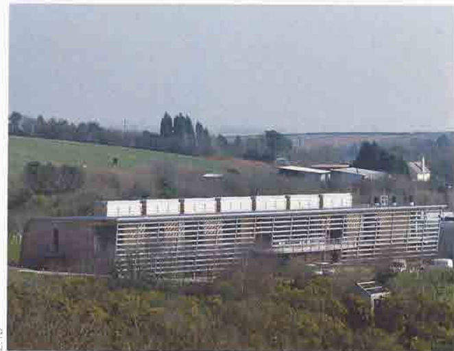
Fig 2.15 General view of the Foundation building Fig 2.16 First floor plan Fig 2.17 Section
