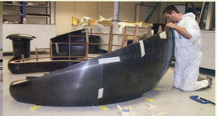
7. Skeleton made from 18mm marine-grade ply components, cut with a CNC router. Finished panels bonded to frame with epoxy to produce rigid shell structure
