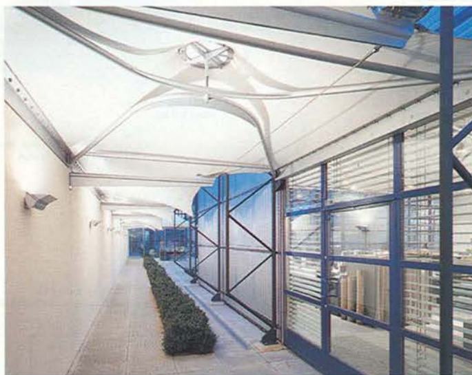
Top: the canopy and glass box form a new entrance. Above: looking back along the reinforced garden wall
