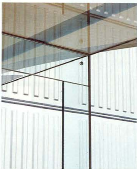
Top: the new canopy provides a sheltered route. Above: detail of structural glass in the reception building
